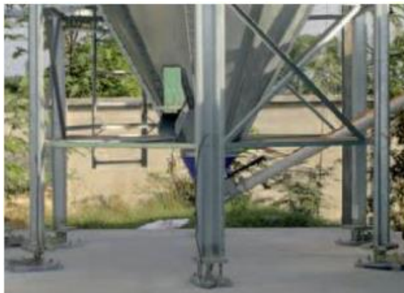
5-rasm. Elektron tenzodatchikda bunkerni tarozida tortish
